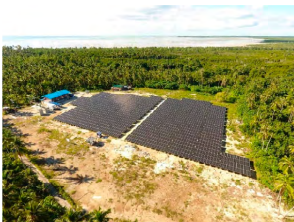
Solar photovoltaic (PV)-diesel hybrid system to improve electricity access, particularly for seaweed-producing communities in the island municipalities of Sitangkai and Sibutu. © Mindanao Development Authority
