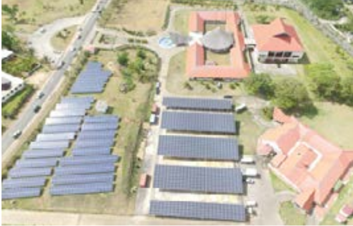
Completed Parliament Buildings: car park and ground-mounted solar PV plants
