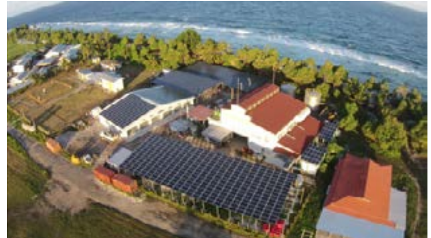
Completed structures with solar PV panels on roofs
