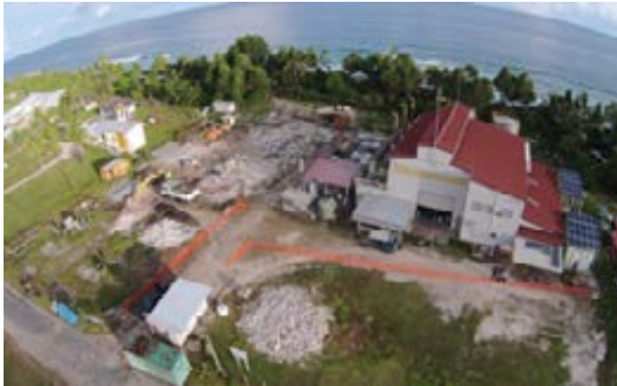
Pre-construction (diesel power station site)
