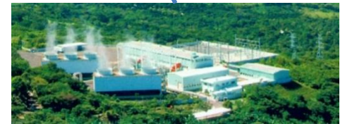
Generation Plant in Berlín 109.4MWe
