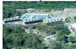
Generation Plant in Ahuachapán 95 MWe
