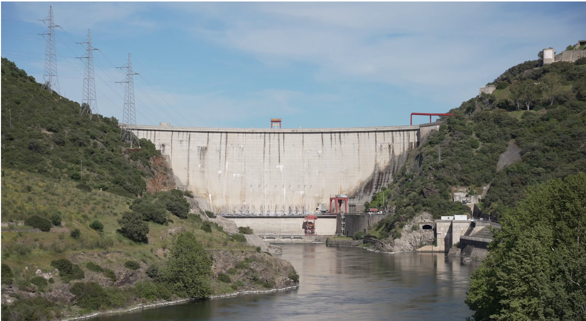
Figure 11 Iberdrola's Torrejón-Valdecañas complex (including hybrid battery storage), Spain
