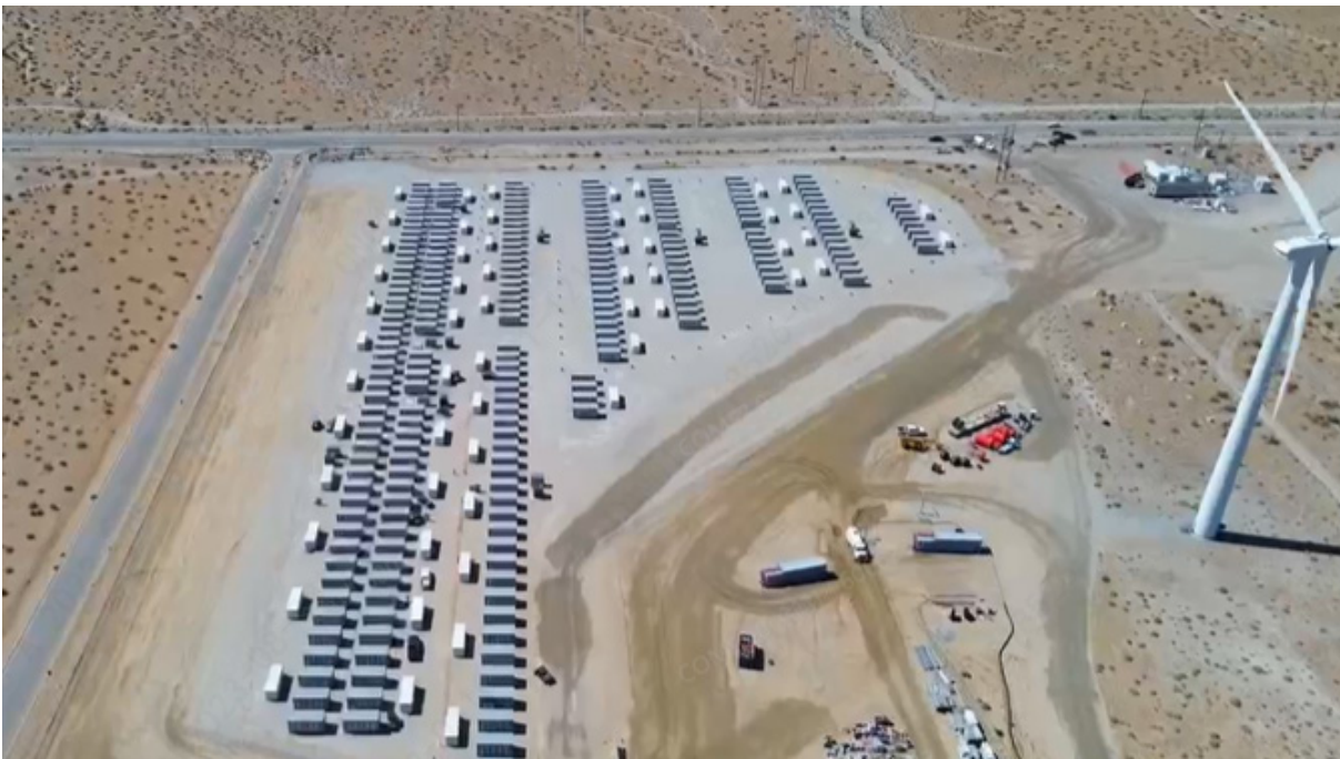
Figure 12 CATL's Desert Peak energy storage project, United States
