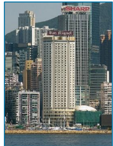
Excelsior Hotel, Hong Kong, one of several hotels using seawater air conditioning
