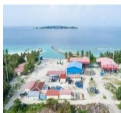
**Small scale waste to energy project, Maldives:** The project includes the construction of waste-to-energy plants on two islands (Addu and Vandhoo). The Vandhoo Island plant has been completed and is handling waste from 40 surrounding islands. It has a generation capacity of 500kW. These waste-to-energy facilities are part of the country's broader waste management framework and contribute to the government's "Scaling Up Renewable Energy Program".
