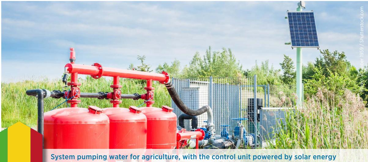
System pumping water for agriculture, with the control unit powered by solar energy
