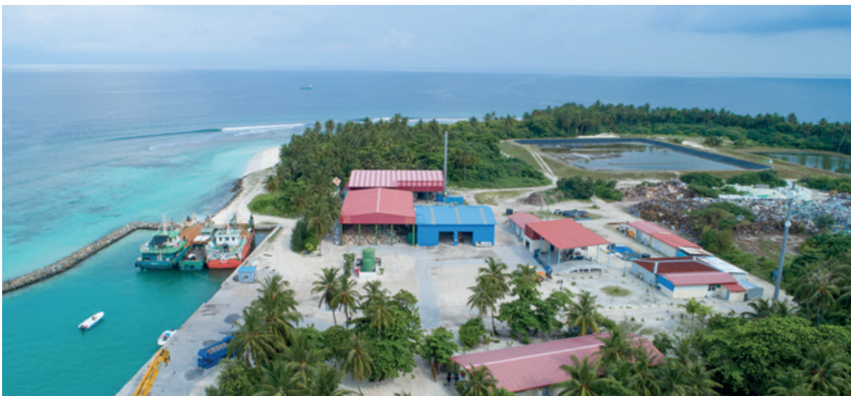
R. Vandhoo island waste to energy facility in the Maldives selected in the first cycle through the IRENA/ADFD Facility Photograph: Ministry of Environment and Energy of the Maldives
