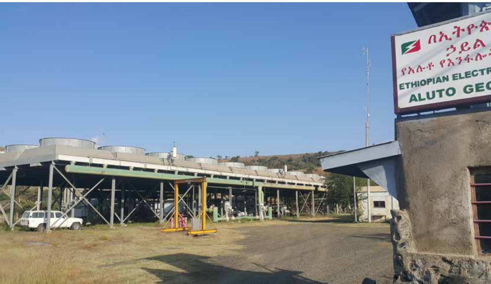
Photograph 1: Aluto-Langano geothermal power plant
