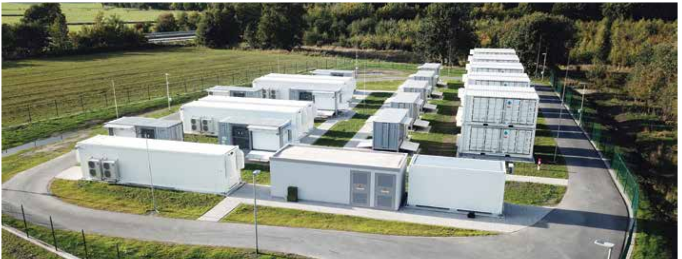
Figure 53: NaS batteries from NGK in Varel (Germany), similar to the ones in Campania region
