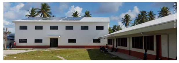
Figure 7. Chuuk school using standalone solar PV with battery storage
