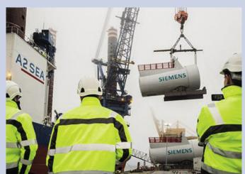
Figure 24: Loading a turbine nacelle aboard an installation vessel
