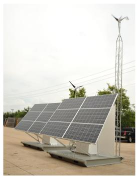
**Figure 7-11-** Two skid-mounted autonomous power units employing solar and wind systems and battery storage.
