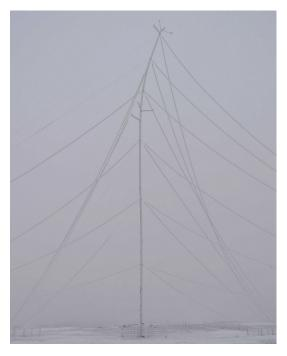
**Figure 12-6** Tower failure caused by heavy icing. (Source: AWS Truepower)
