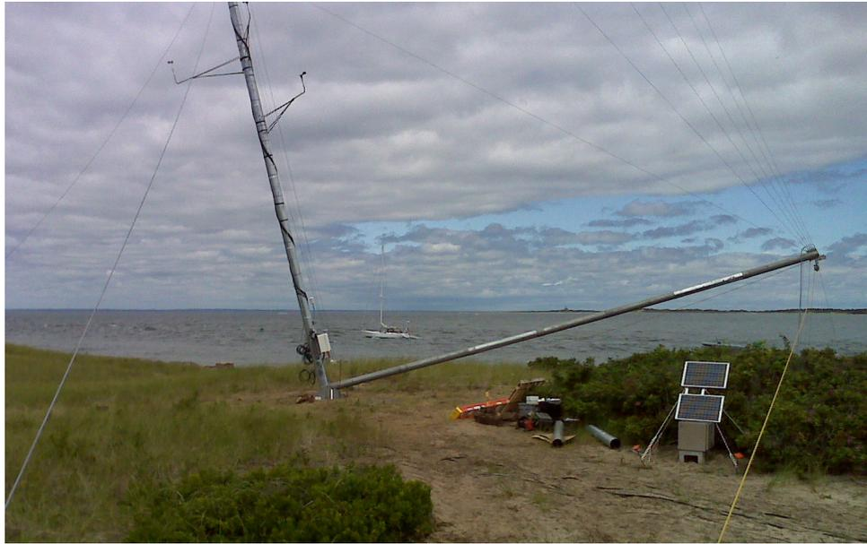
**Figure 9-5** Tilt-up meteorological tower being raised with a gin pole. (Source: AWS Truepower)
