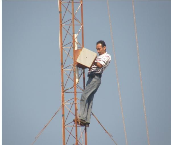
**Figure 9-1** Unsafe climbing practices like those shown here are a serious danger to personnel. In this case, the climber has no head protection, climbing harness, or fall protection. (Source: AWS Truepower)
