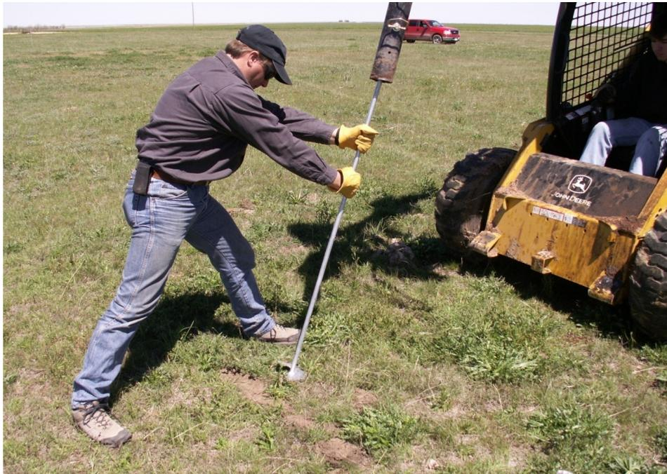
**Figure 9-6** Example of a screw-in guy-anchor installation. (Source: AWS Truepower)
