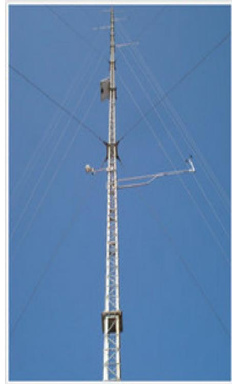
**Figure 7-2** A guyed lattice tower instrumented for wind monitoring. (Source: AWS Truepower)
