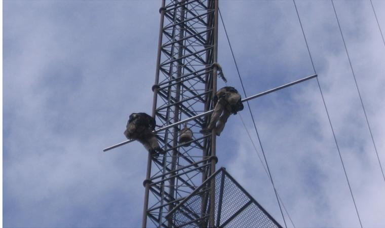
**Figure 9-2** Safe climbing practices are shown here. The technicians are working as a team while employing appropriate personal protective equipment, equipment management, and fall protection. (Source: AWS Truepower)
