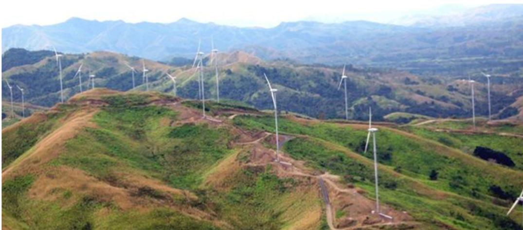
**Figure 5-2** The Butoni wind project on Viti Levu, Fiji. This 10 MW project consisting of thirty-seven 275kW Vergnet turbines illustrates a typical utility-scale project for a large island. (Source: Vergnet.)
