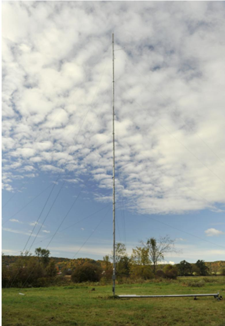
**Figure 7-1.** A 34 m tubular tilt-up tower. (Source: NRG Systems)
