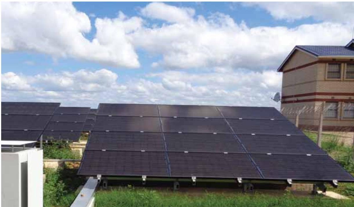
A 32 kW solar array supplies power to the Border Post in Mhlumeni
