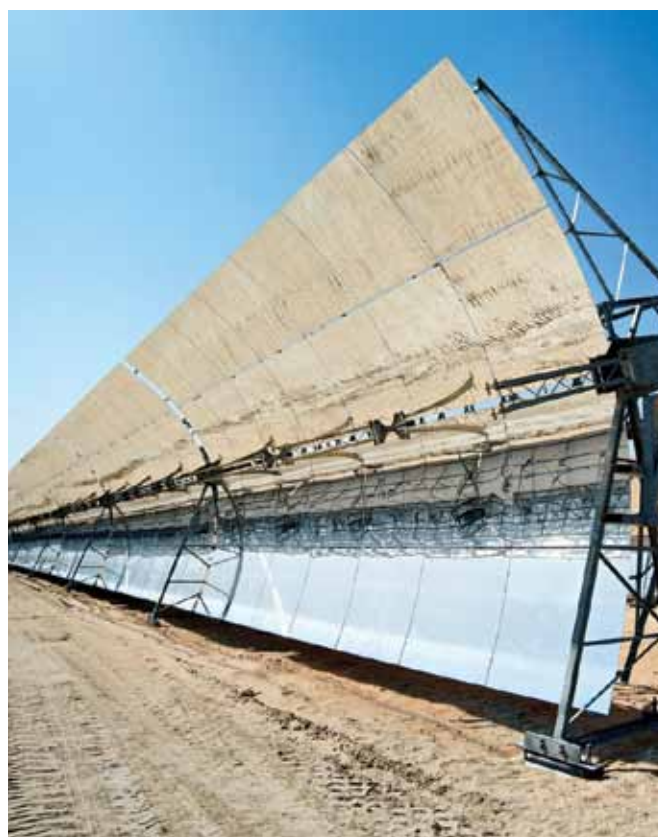
Shams-1- a 100 MW CSP plant in Abu Dhabi Photograph: Masdar
