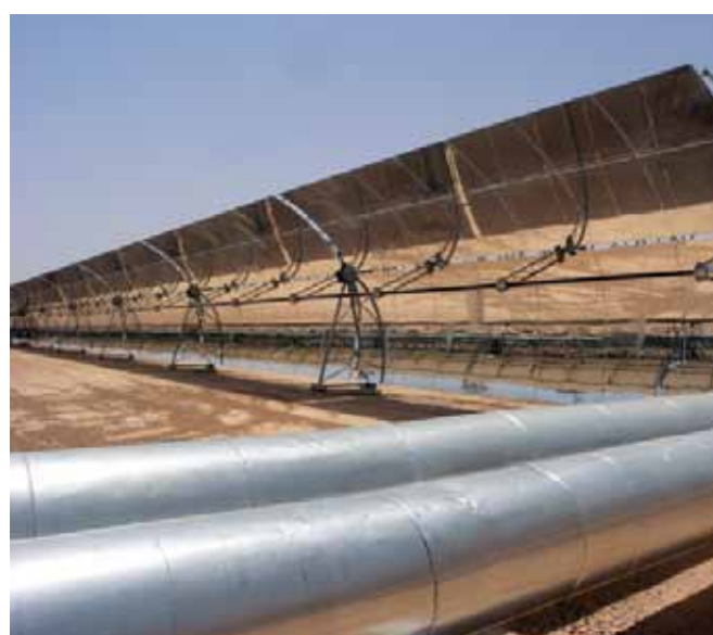
Combined-cycle gas / Concentrated Solar Power 150MW (25MW Solar) Hassi Ramel, Algeria Photograph: RCREEE
