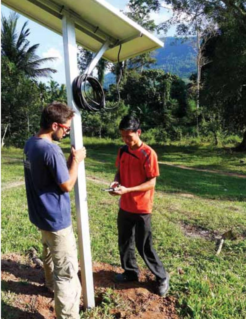
*Installation and orientation of a solar PV panel (ARE)*
