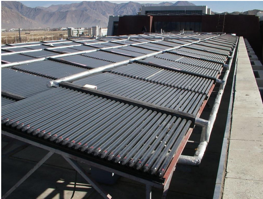
Installation of solar collectors
