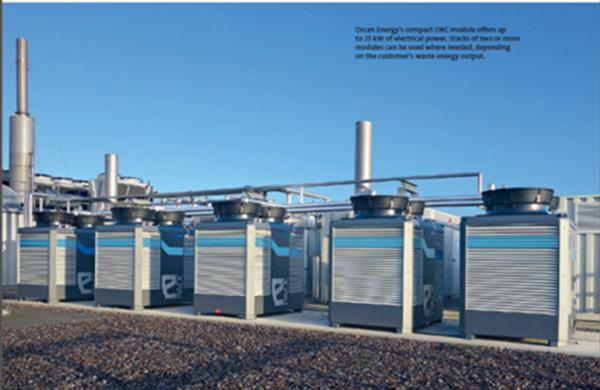
Compact micro power plants turning heat waste into energy!
