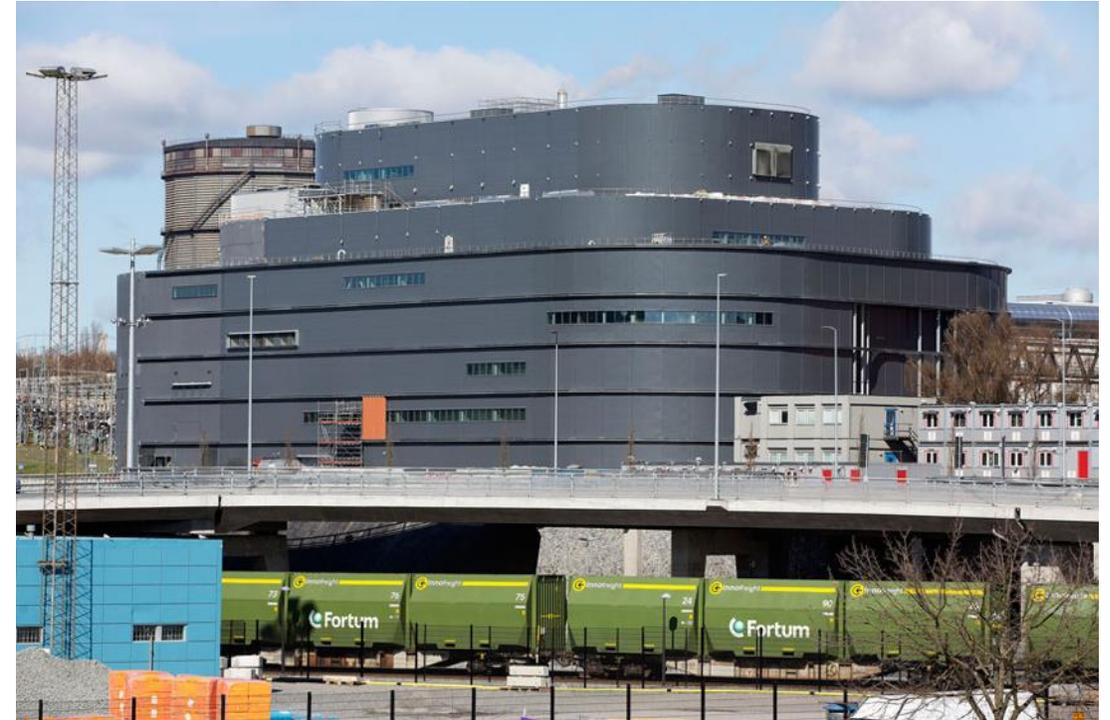
*Värtaverket plant in Stockholm – largest combined heat and power plant. 1.7 TWh heat and 680 GWh electricity. Fuel – wood chips
