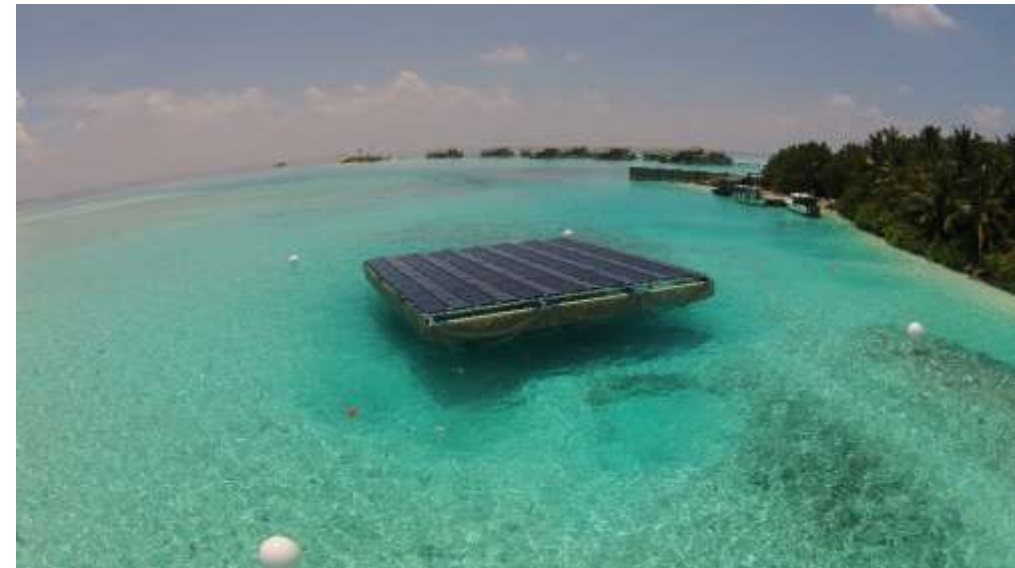
Final system installed - 2015
