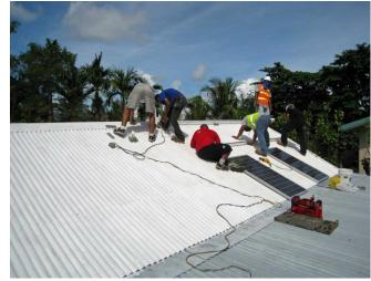
Laying out the panel attachment rails
