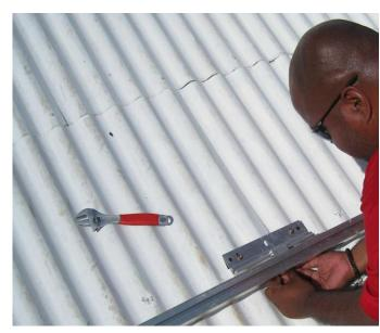
Fastening the rails to the roof
