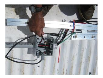
Completing the wiring in the main junction box
