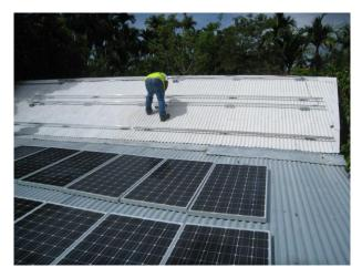
Checking the rail attachments
