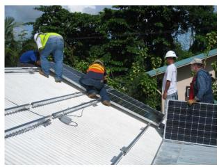
Mounting the panels on the rails
