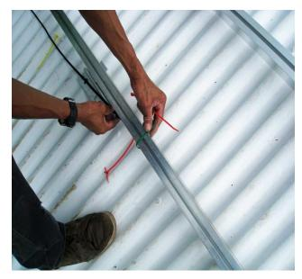
Temporarily tying the wiring to the rails
