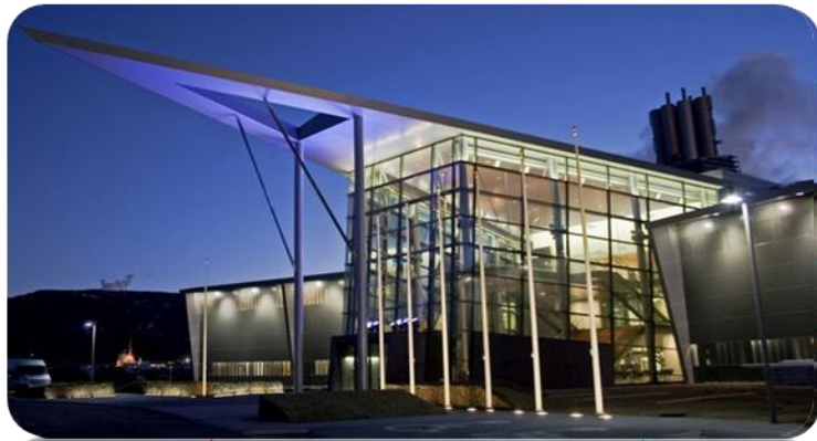
Hellisheidi Geothermal Power Plant
