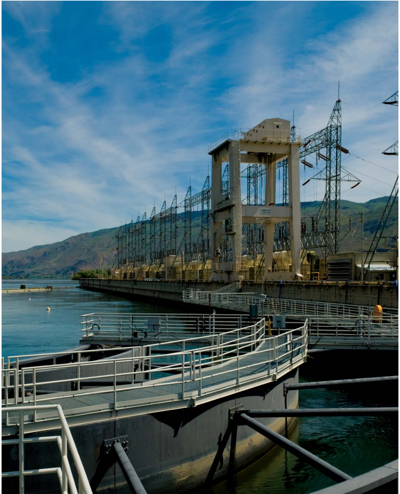
Hydropower plant Photo Courtesy: Shutterstock
