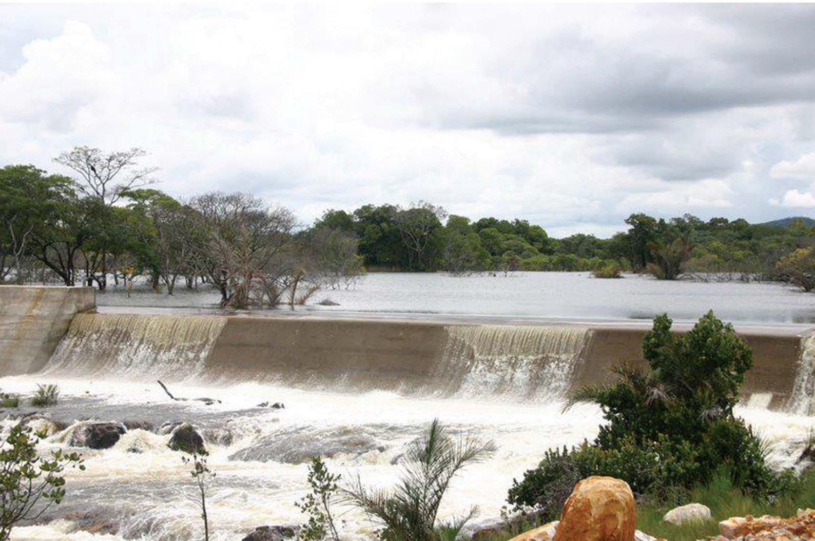
Mini-hydro dam on the Nanshya River, Zambia Courtesy: REA
