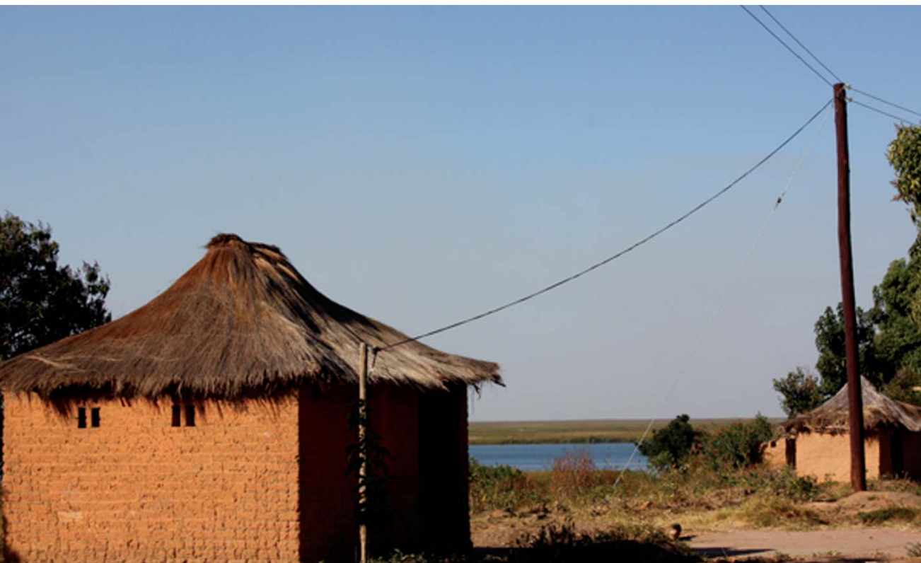
Decentralised rural electrification grid Courtesy: REA
