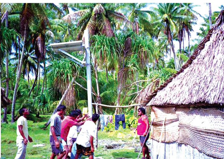
Installing a solar panel in a Kiribati home
